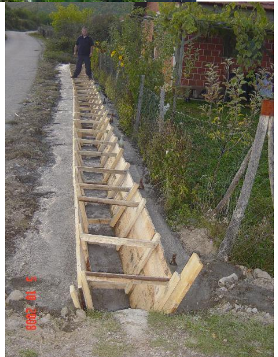
Irrigation channels in Brestovik village donated by UNDP project
